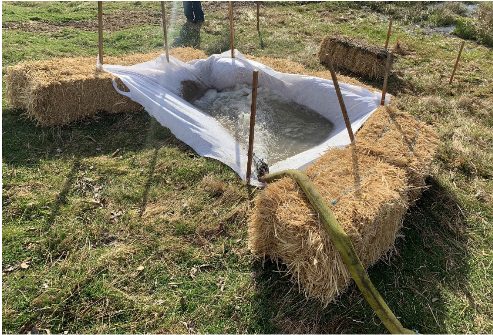
Figure 5: Standard Installation of Geofabric Filter Dam
