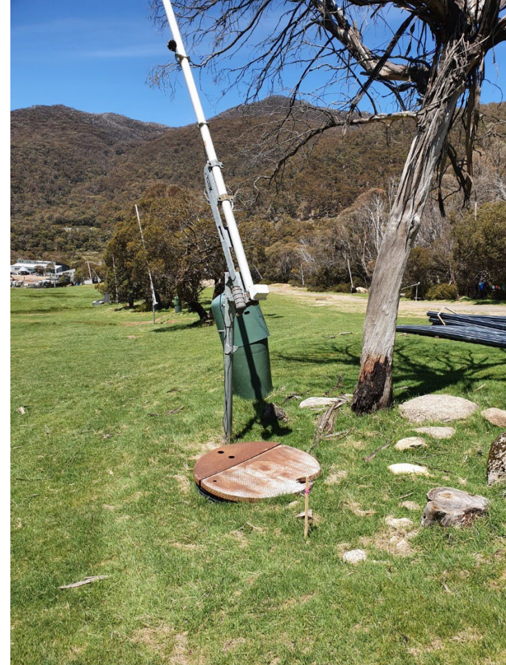
Photo A5: TT10 #3 (Easy Does It, skiers right) – replacement of existing lance gun with TT10 fan gun
