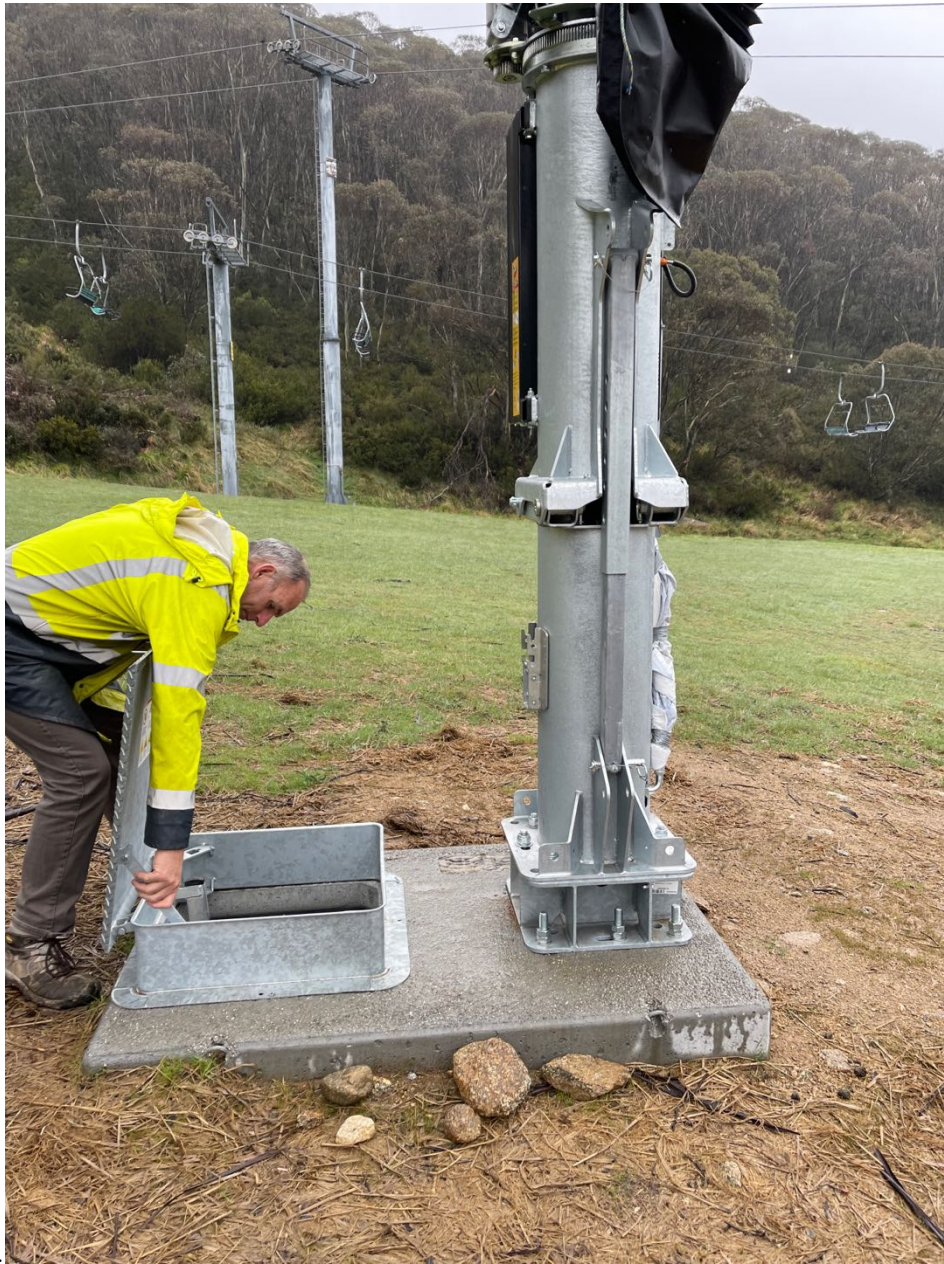
Photo 7 Example of snowmaking gun on top of concrete pit
